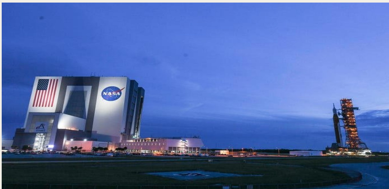
Plate 4. Kennedy's Vehicle Assembly Building — a different house on the same coast. Crew-13 is posted for SLC-40, not LC-39B.
