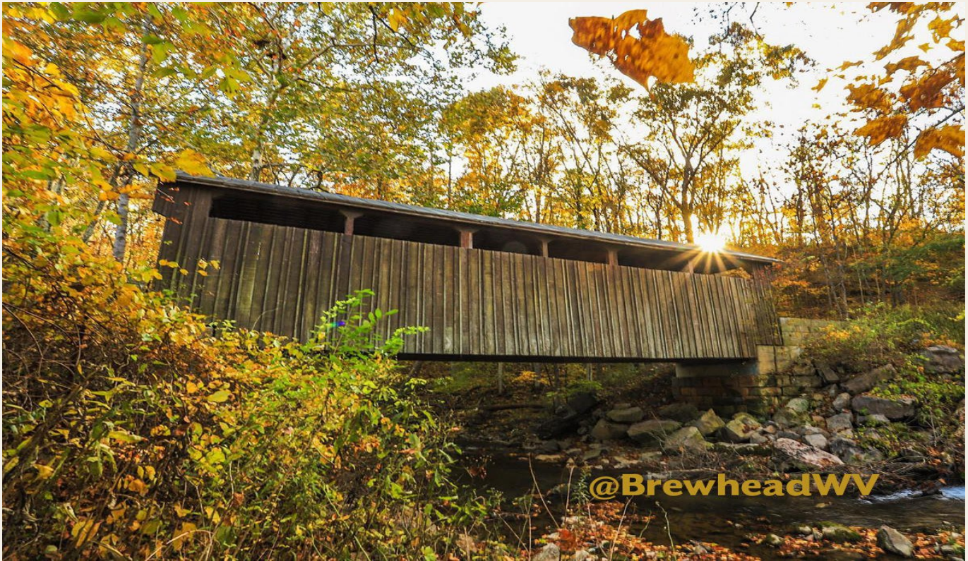
Plate 5. Greenbrier Valley cover — local water and timber, not the project limits. The work named in Call 011 is asphalt on U.S. 219 from Renick toward the Pocahontas line.
